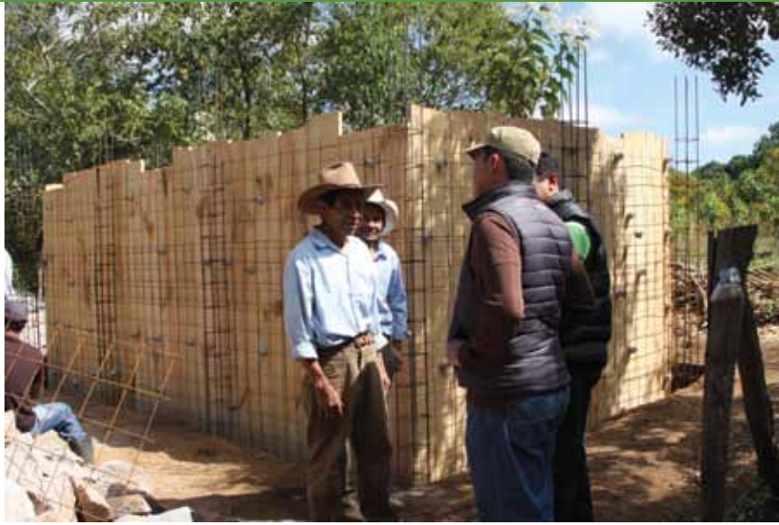
Project Manager and Engineer at site of water distribution tank
