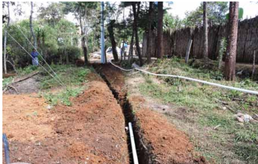
Installing a new water system
